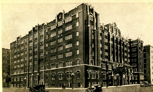
NEW Y.M.C.A. BUILDING, COLUMBUS, OHIO.
